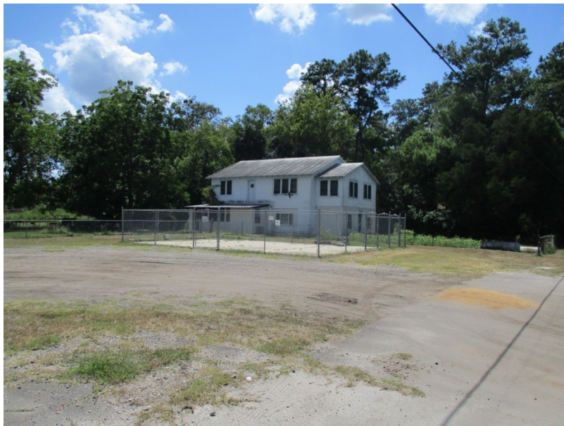
Vacant commercial structure in the southwest quadrant.
